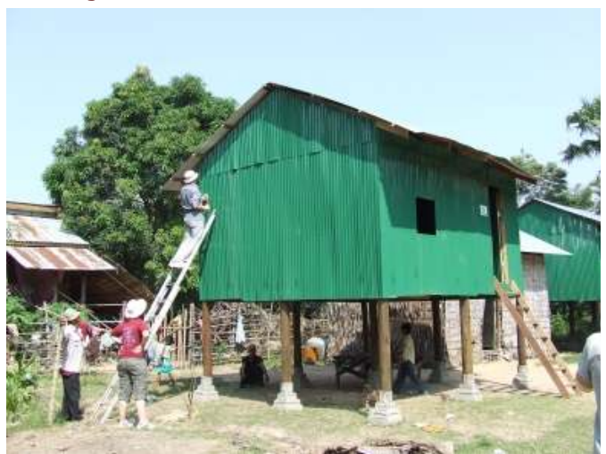
Building houses in Takeo Province
