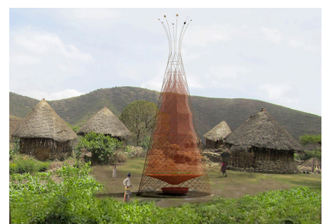
The Warka Water Tower can produce over 25 gallons per day for remote villages
